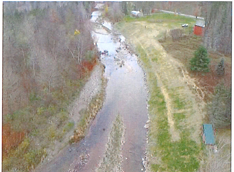
Regraded bank with stone toe, before plantings
