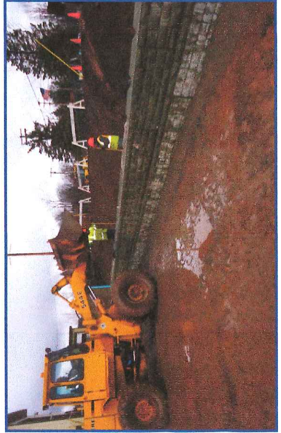
County Forces Installing a V-Lock Designed Block
