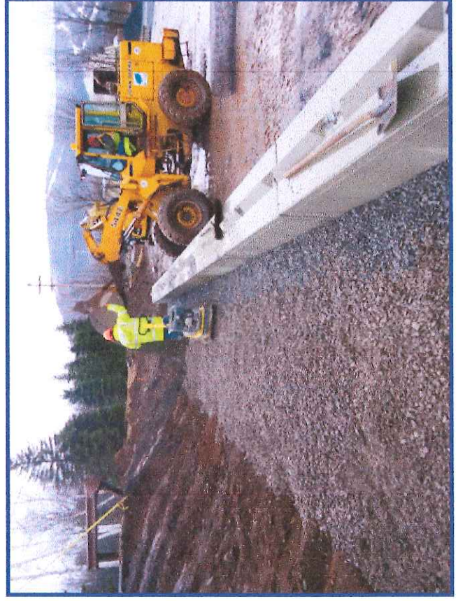
County Forces Installing a V-Lock Designed Block
