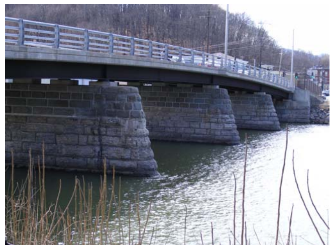
The Uncle Sam Bridge limits boat navigation to the upper part of the Catskill Creek harbor with only 15' of clearance at low tide and as little as 10' at high tide.
