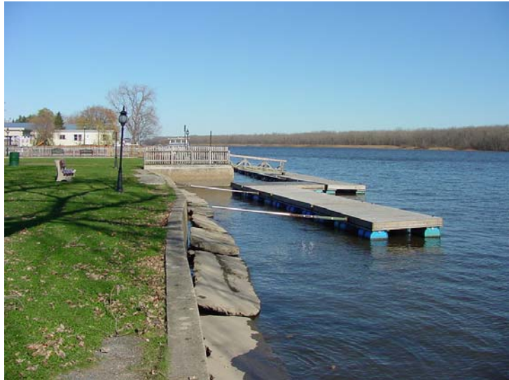
Old wooden and concrete bulkheads will be replaced with steel piling. New docks as well as a wide waterfront promenade will be constructed.
