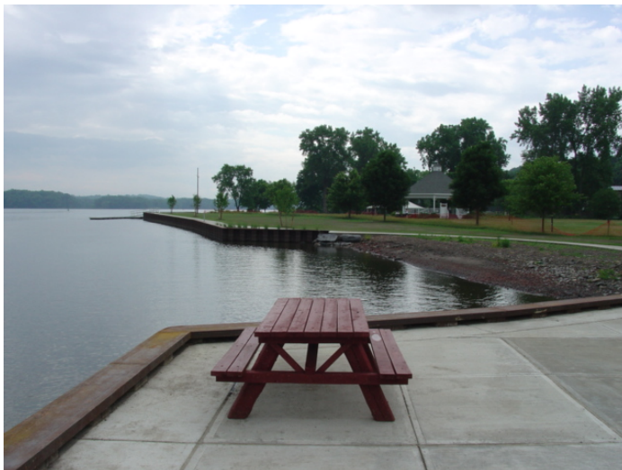
Rehabilitation of the Riverside Park shoreline included extensive bulk-head replacement as well as provision of a softer shoreline that allows passive access to the rivers edge.
