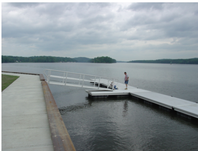
A new steel bulkhead, concrete promenade and modern lightweight docks were primary components of the parks recent rehabilitation
