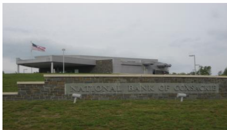
The National Bank of Coxsackie is one of the two bank buildings recently constructed on the "Eastern Gateway."
