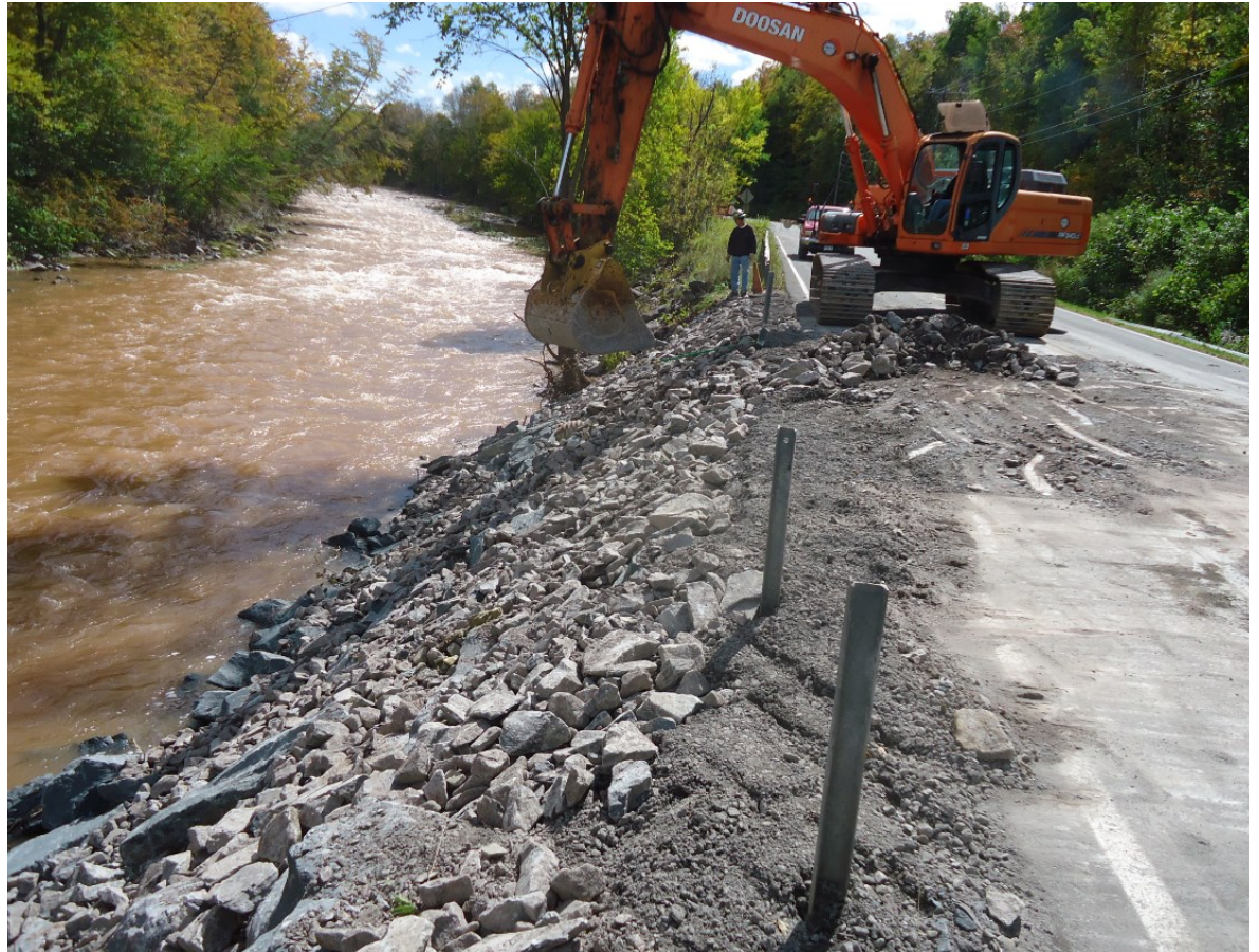
Cr. 83 (Ski Bowl Road) - Slope Stabilization Before & During.
